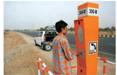
Emergency call box on NH-8
